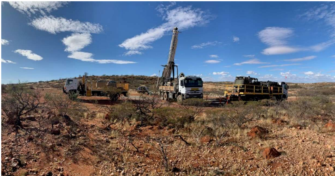
Figure 1: One of the drill rigs on site
